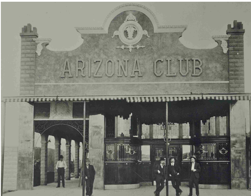
Figure One. The Arizona Club ca. 1909. This photo shows the building's original façade. UNLV Libraries, Special Collection.
